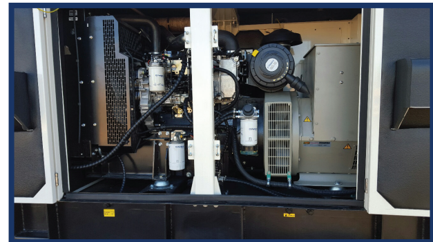
EASY ACCESS FOR MAINTENANCE
