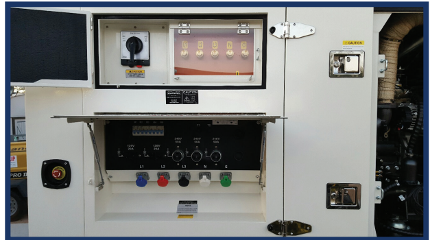
CUSTOMER CONNECTION PANEL
