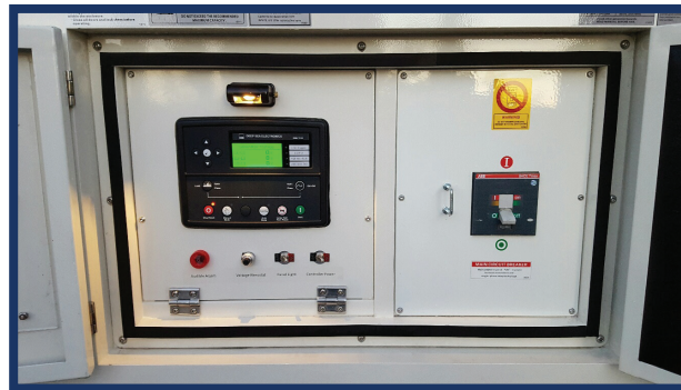
REAR CONTROL PANEL WITH MLCB
